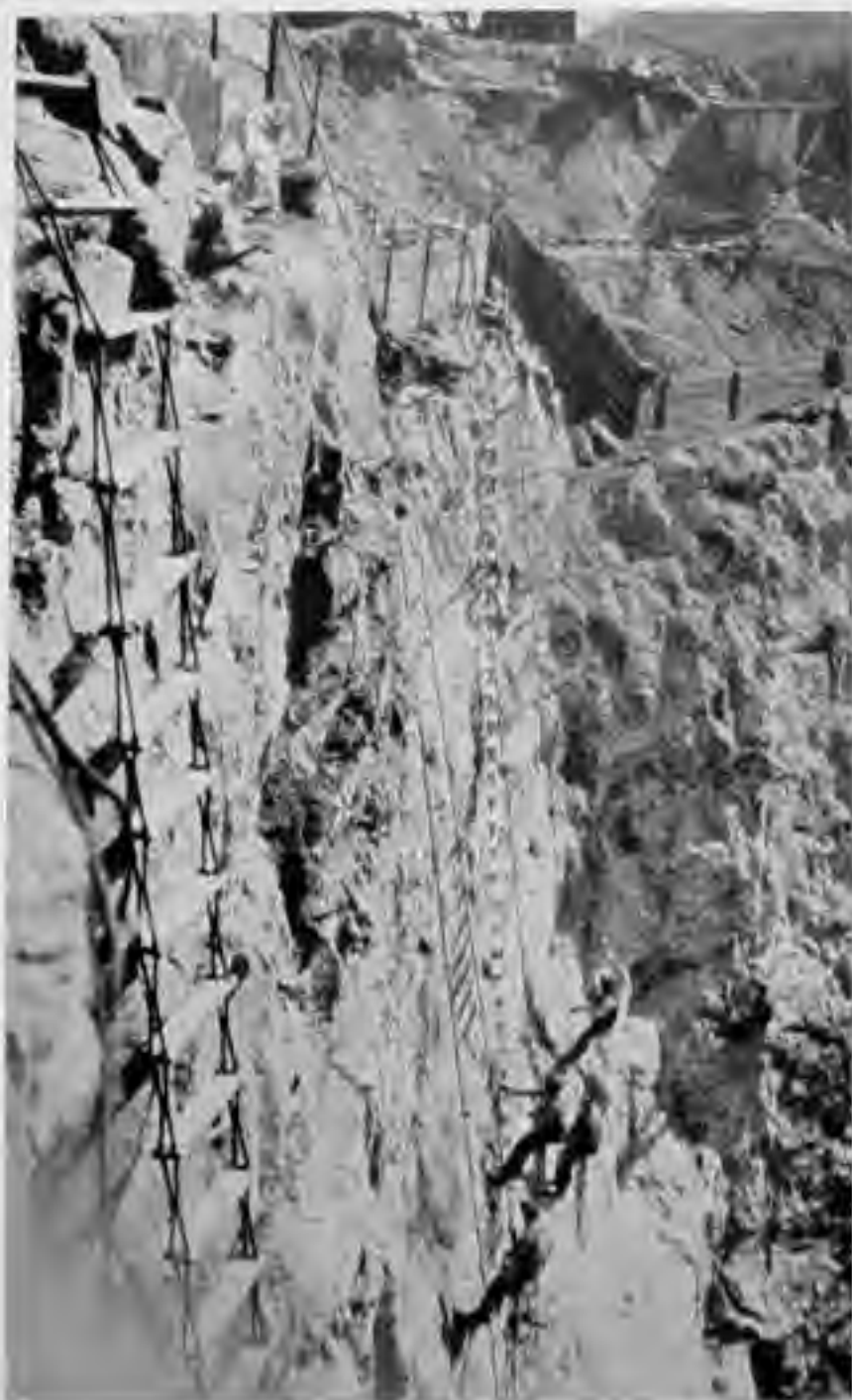
FIG. 11. Mining for cryolite at Isigot, Greenland. Blasting to the open; drilling holes for explosive with pneumatic drills.
